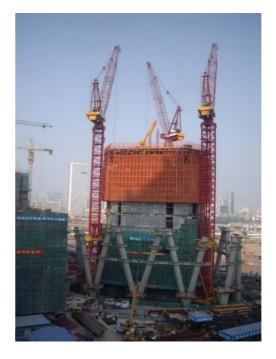
Figure 44. Climb-form system of central core.
