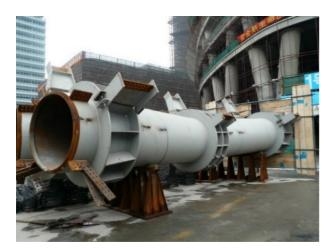
Figure 45. Prefabricated diagrid steelwork.
