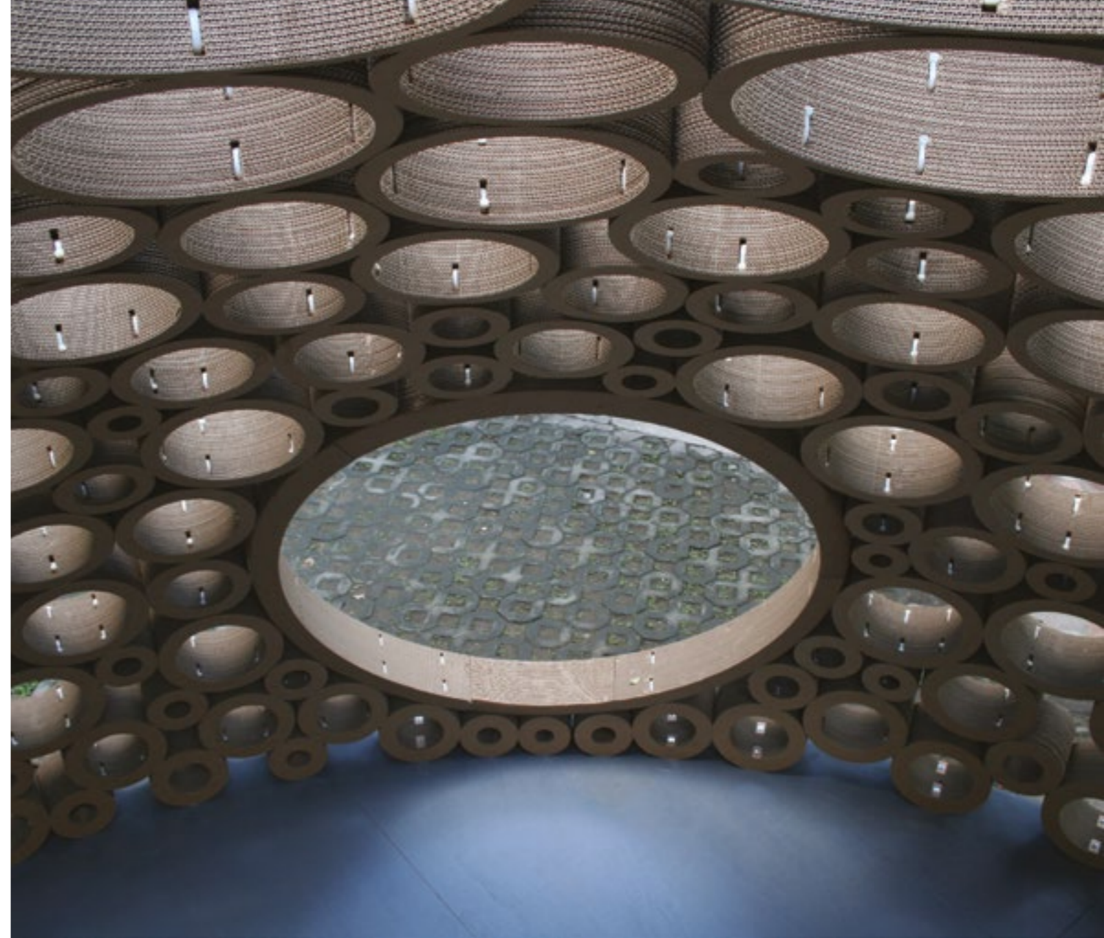
Paked Pavilion , Shanghai, 2010. Progetto di Min-Chieh Chen, Michele Leidi e Dominik Zausinger (CAAD ETHZ), con la collaborazione di Jeannette Kuo e la supervisione di Tom Pawlowsky. Packed pavilion . Shanghai, 2010. Project by Min-Chieh Chen, Michele Leidi and Dominik Zausinger (CAAD ETHZ), with the collaboration of Jeannette Kuo and supervised by Tom Pawlowsky.
